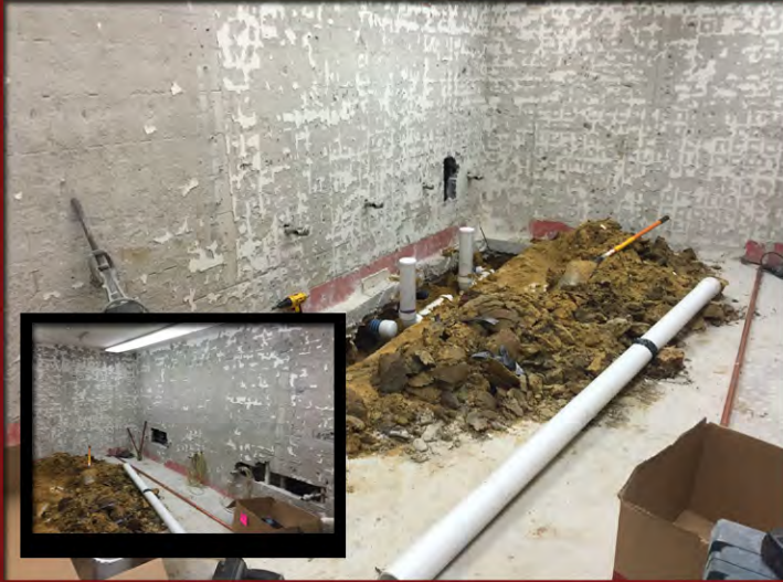
Demolished restroom plumbing and finishes.
