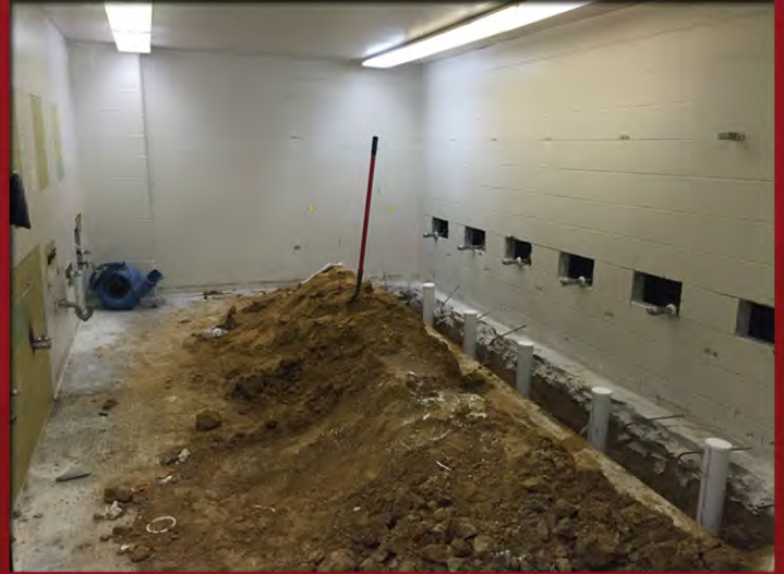
Began installing new plumbing piping.
