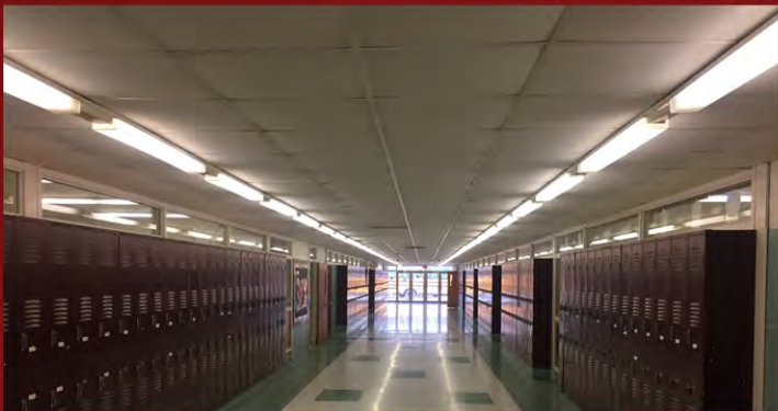
Installed new ballast and modified lamps at corridor lights.
