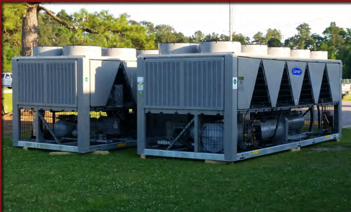
Received delivery of the chillers.
