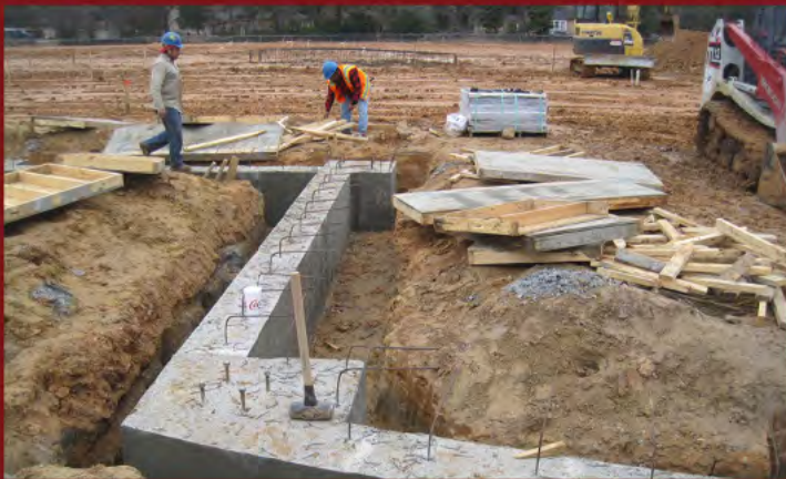
Installing underslab plumbing and grade beams.
