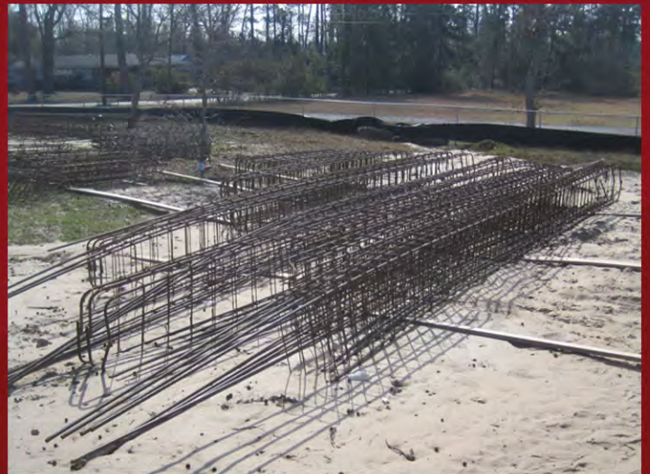
Area A steel and grade beam reinforcement awaiting installation.
