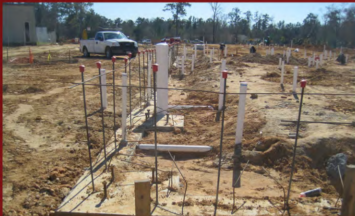
Area A steel and grade beam reinforcement awaiting installation.
